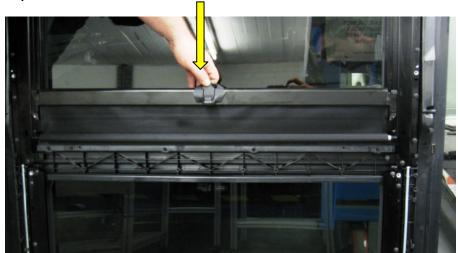
5. Dis-assemble blind's rotator side from mounting point by pulling the rollo tube away from the rotator mounting.
